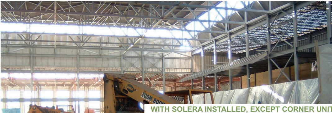
WITH SOLERA INSTALLED, EXCEPT CORNER UNIT
