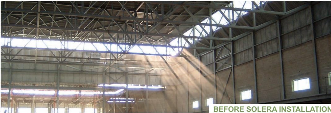
BEFORE SOLERA INSTALLATION
