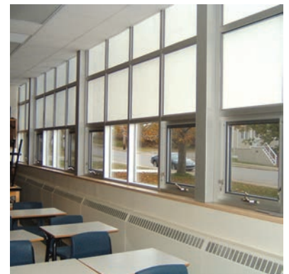
Installing Solera® above the vision glass units dramatically cuts back glare, converting it to soft, well-distributed diffuse daylight.
